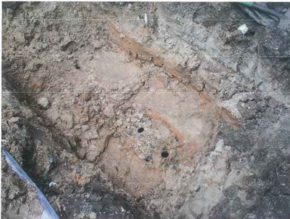
Picture 2: UST 453Elderberry excavation in progress.
